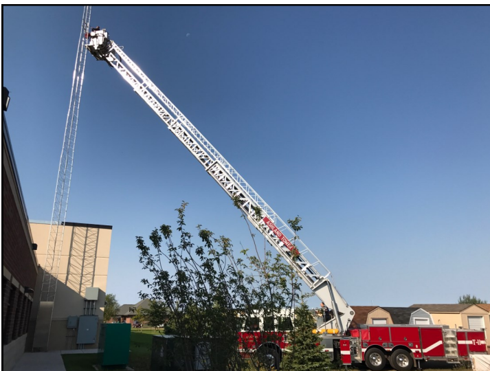
Repair to Communications Tower
